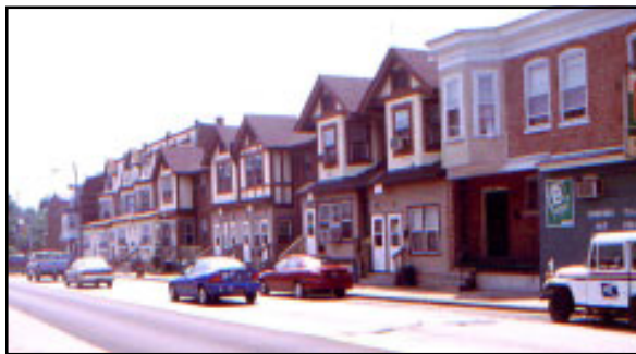
Figures 3.7-3.9. Many sections of the Village's main streets give a negative impression of the area. This gas station on Market (top) has been closed for years; Vandever Avenue (middle photo) is the least attractive; and Concord Avenue has fewer problems, but could still improve.
