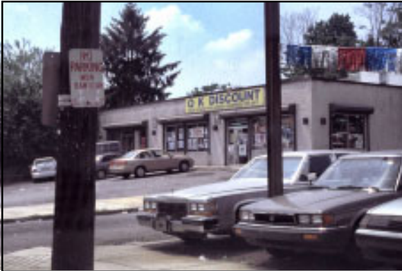
Figure 3.10-3.11: Buildings on Market Street. The top photo shows structures built as residential but no longer suited for residential or for adaptation to commercial. The bottom photo shows a more recently-built convenience store that is poorly maintained and has so many signs posted in the windows that you can no longer see into the store.
