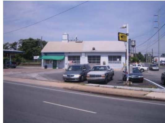
Gas station on Northeast Boulevard in the C-5 district
