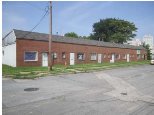
Vacancy and underperforming auto repair shops on 13th Street
