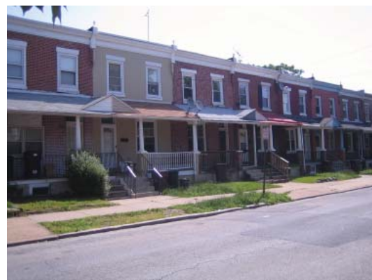
Rowhouses on 17th Street in the R-3 Zone
