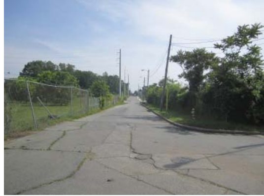
14th Street Rail Spur located in the floodplain
