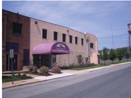
Existing New Destiny Fellowship Church building
